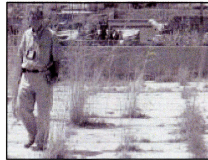
Jim Peak inspects the leaky roof of a school in Dahuk, Iraq.
